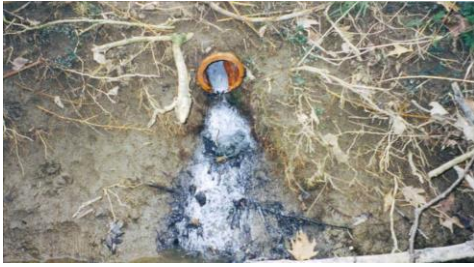
Sewage draining into a ditch is a significant public health hazard.
